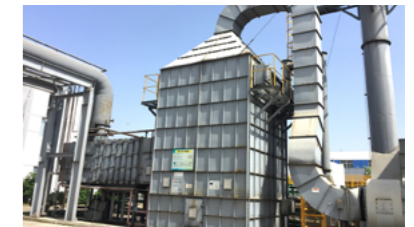
FEDZ installed the smoke purification system
