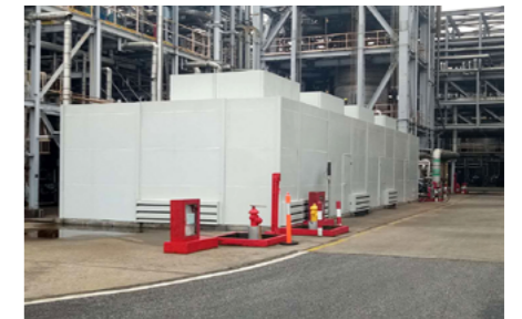
OPSC installed acoustical barrier around equipment.
