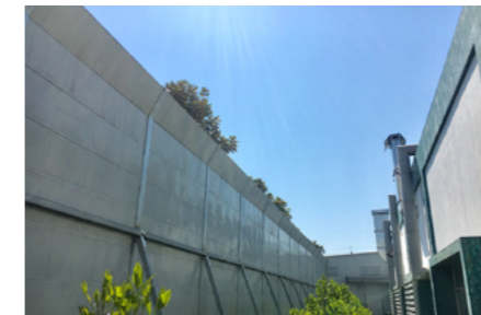
FEIS installed acoustical barrier around equipment.
