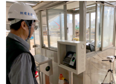
Using Smart Technology for Construction Site Management
