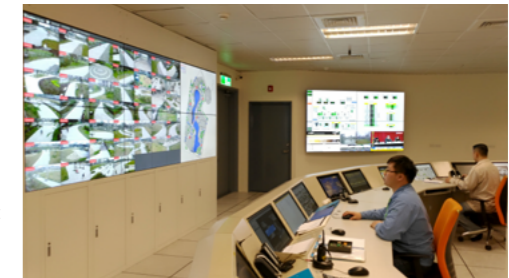
Tpark Disaster Prevention Center
